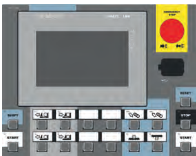
CONTROL PANEL: SIEMENS (X-CNC)
